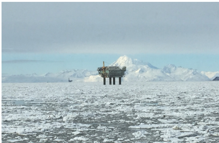
Figure 3. Cook Inlet drilling rig.
